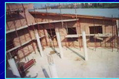
Pilastri e travi in c.a.
