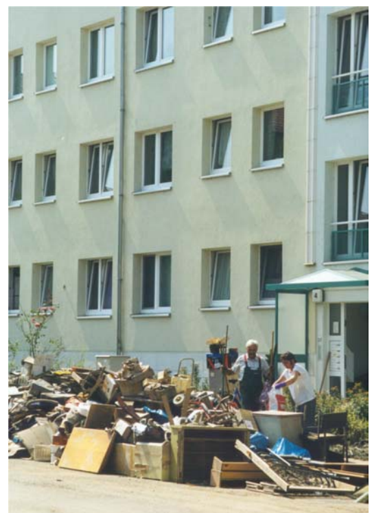
Contents damage in an apartment block in Dresden
