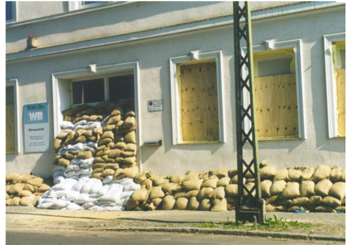
Waiting for the flood: Sandbag and wooden board protection of property in an evacuated area of Magdeburg
