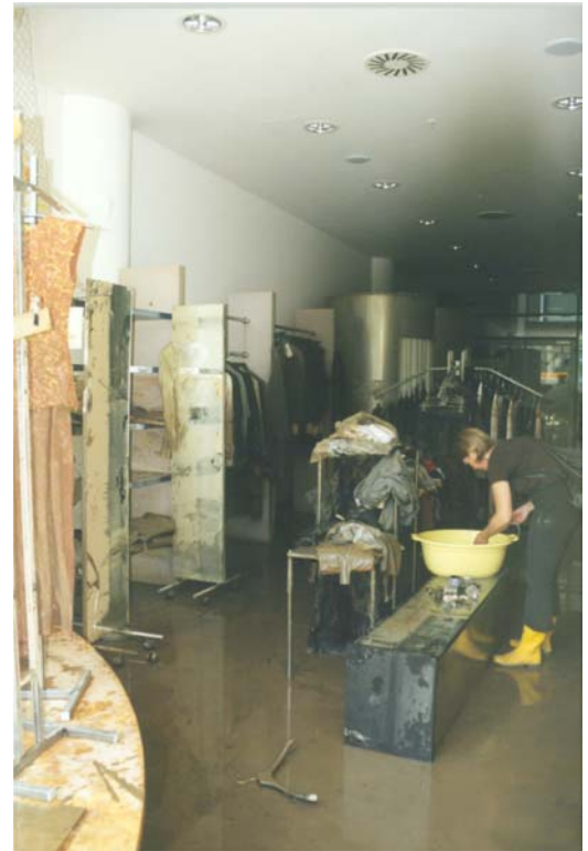
Contents damage to clothing store in Dresden
