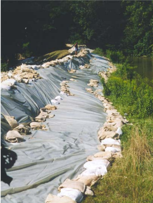
River dyke heightened with polythene and sand bags outside Dessau, downstream from Dresden. This defence held, saving a residential district and part of the town centre behind the defence
